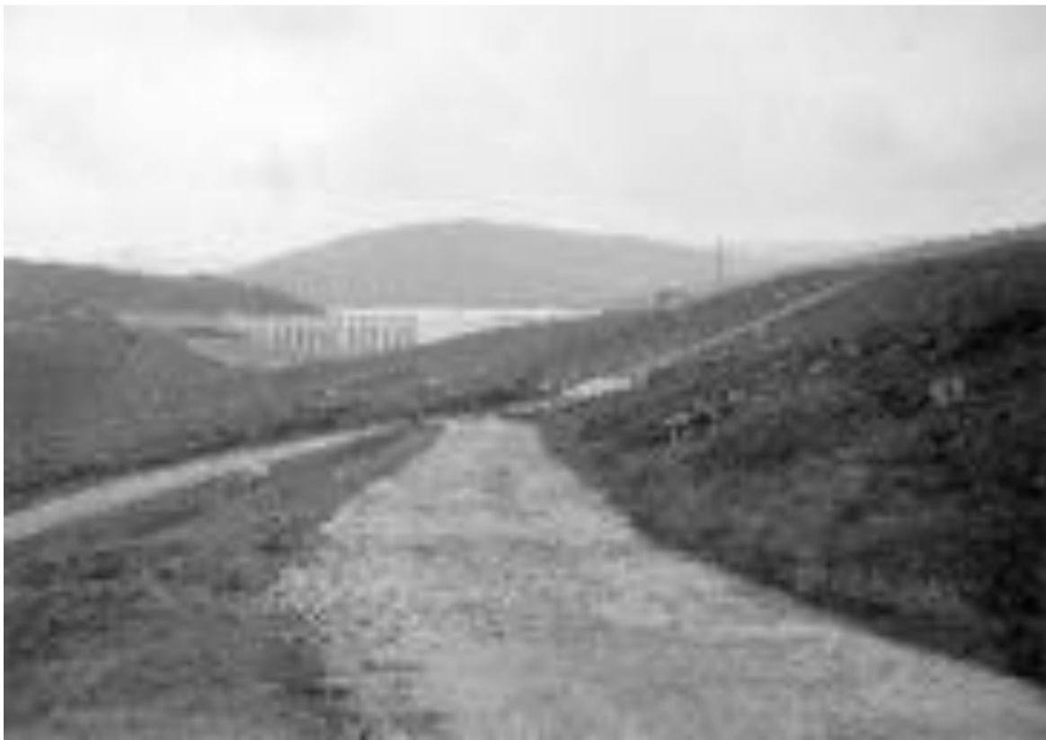
The new Loch Rannoch, a reservoir, just about finished
